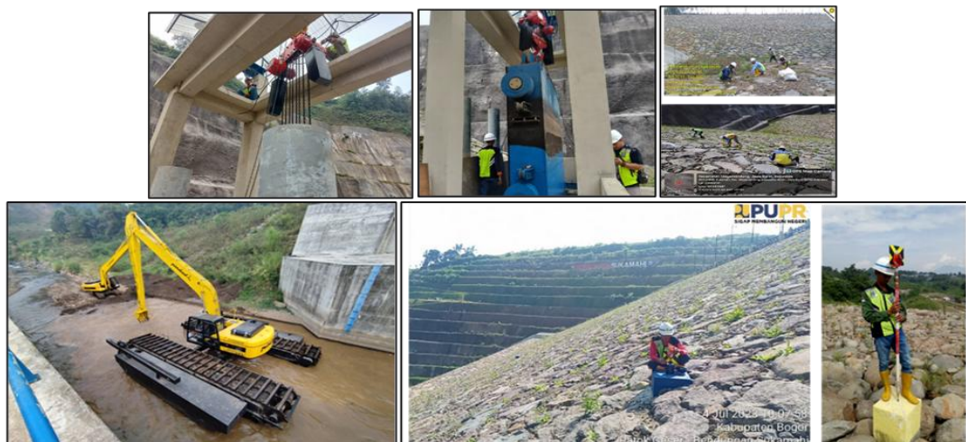
Figure 2. Operational, Maintenance, and Monitoring Activities of the Sukamahi Dry Dam
